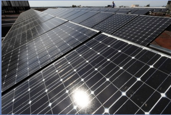
Rooftop Solar Panels
