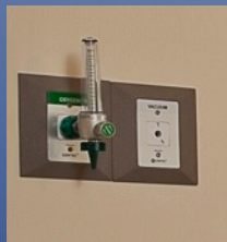
Oxygen system without tank delivery
