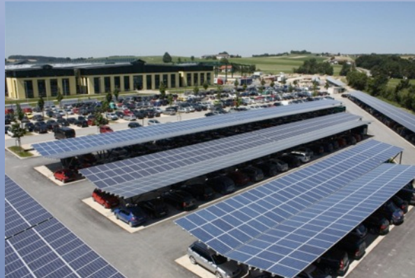
Carport/Garage Solar Panels & preferred parking for efficient cars
